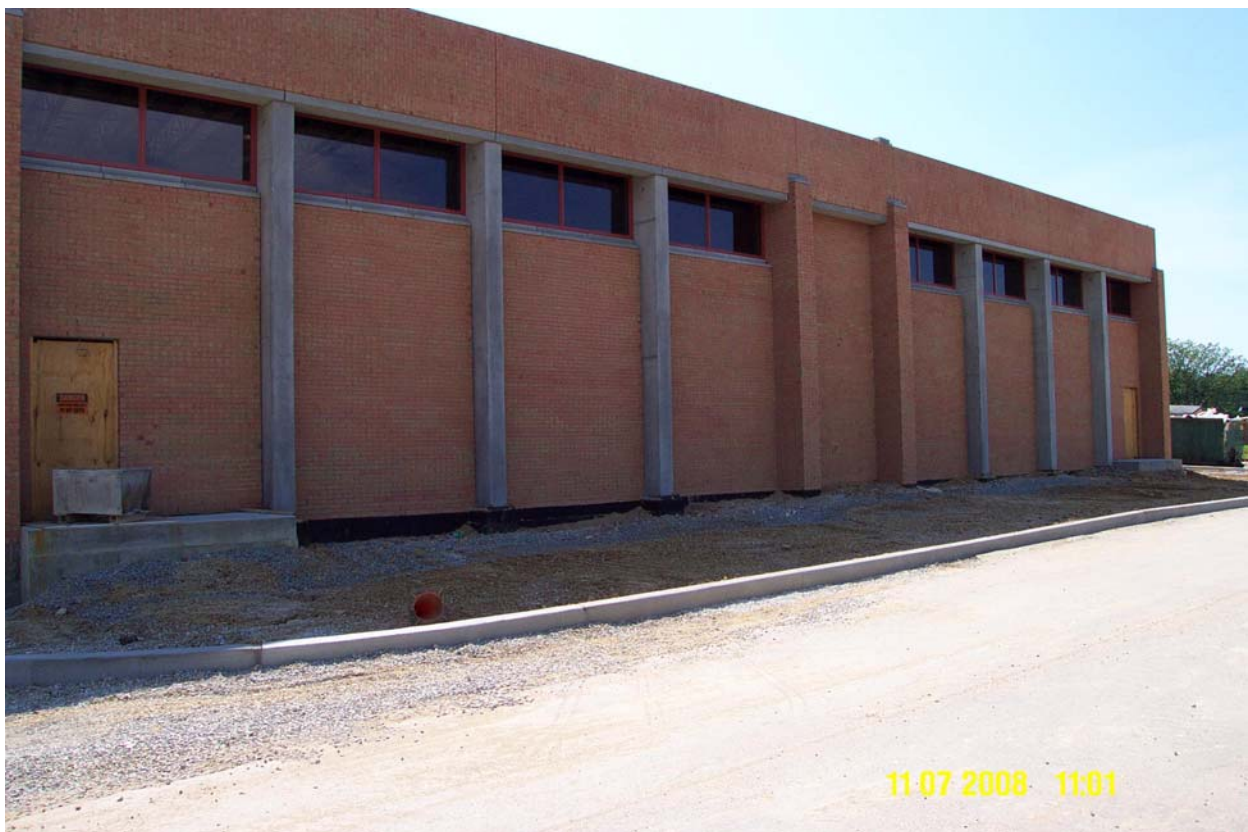
Figure 16 and 17: Original above, additions below
