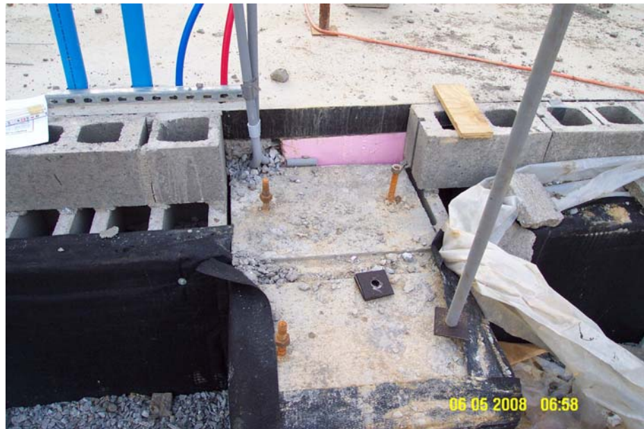
Figure 19: Column anchor system to foundation
