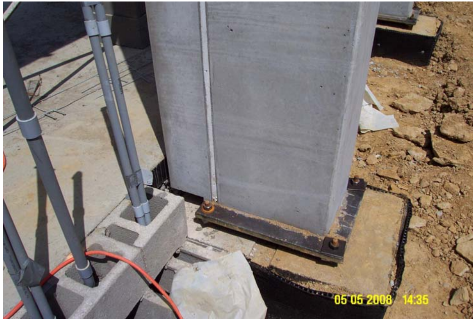
Figure 20: Precast columns on base plate anchored to foundation
